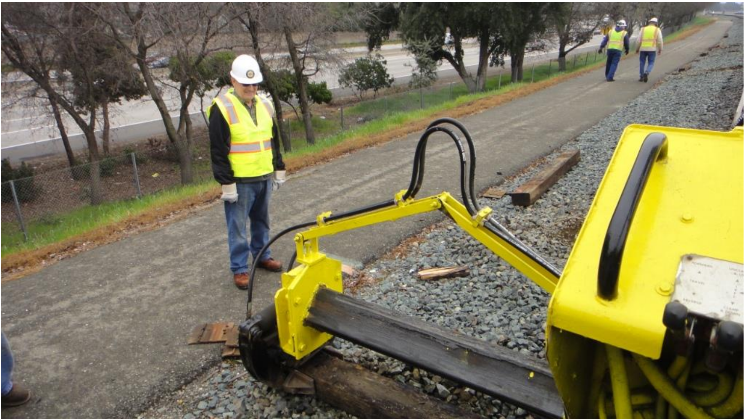
Mike W. is very impressed with the way the 125 whips rotten ties out from under the track
