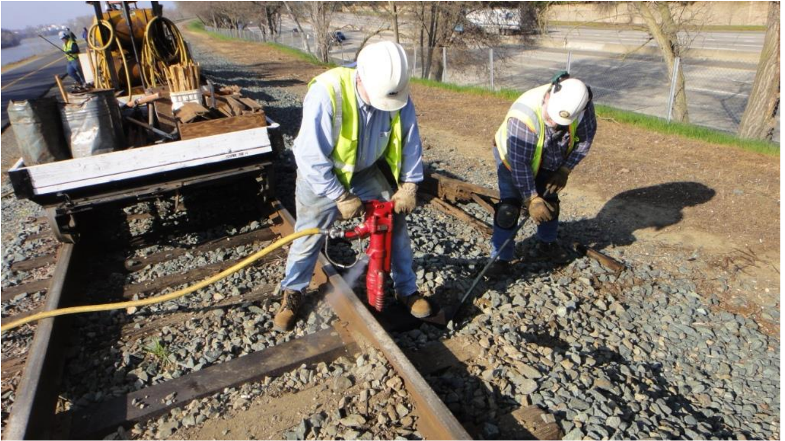
Mike M. drives a spike with the pneumatic spiker as Frank nips-up the tie
