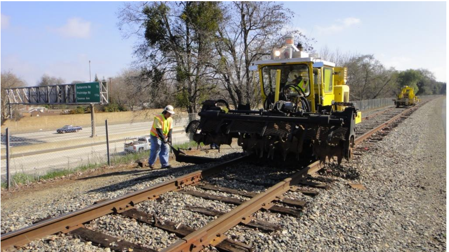
Alan operates the scarifier while Mike F. uses the inserter function to pull in a new tie
