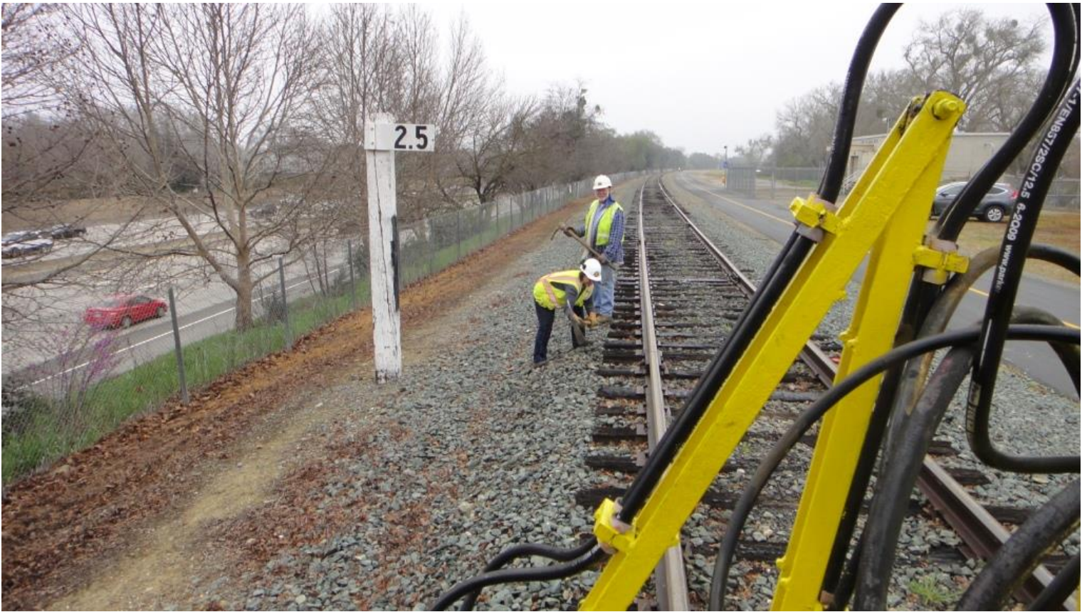
Pam, our Designated Supervisor of the Mattocks Tool (DSMT), and Mike M. dig out the tie-ends so that the 125 can grab them easier
