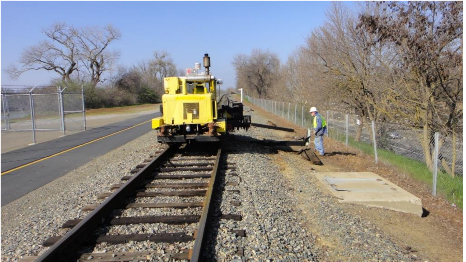
Mike M. places a new tie using the inserter function on the scarifier
