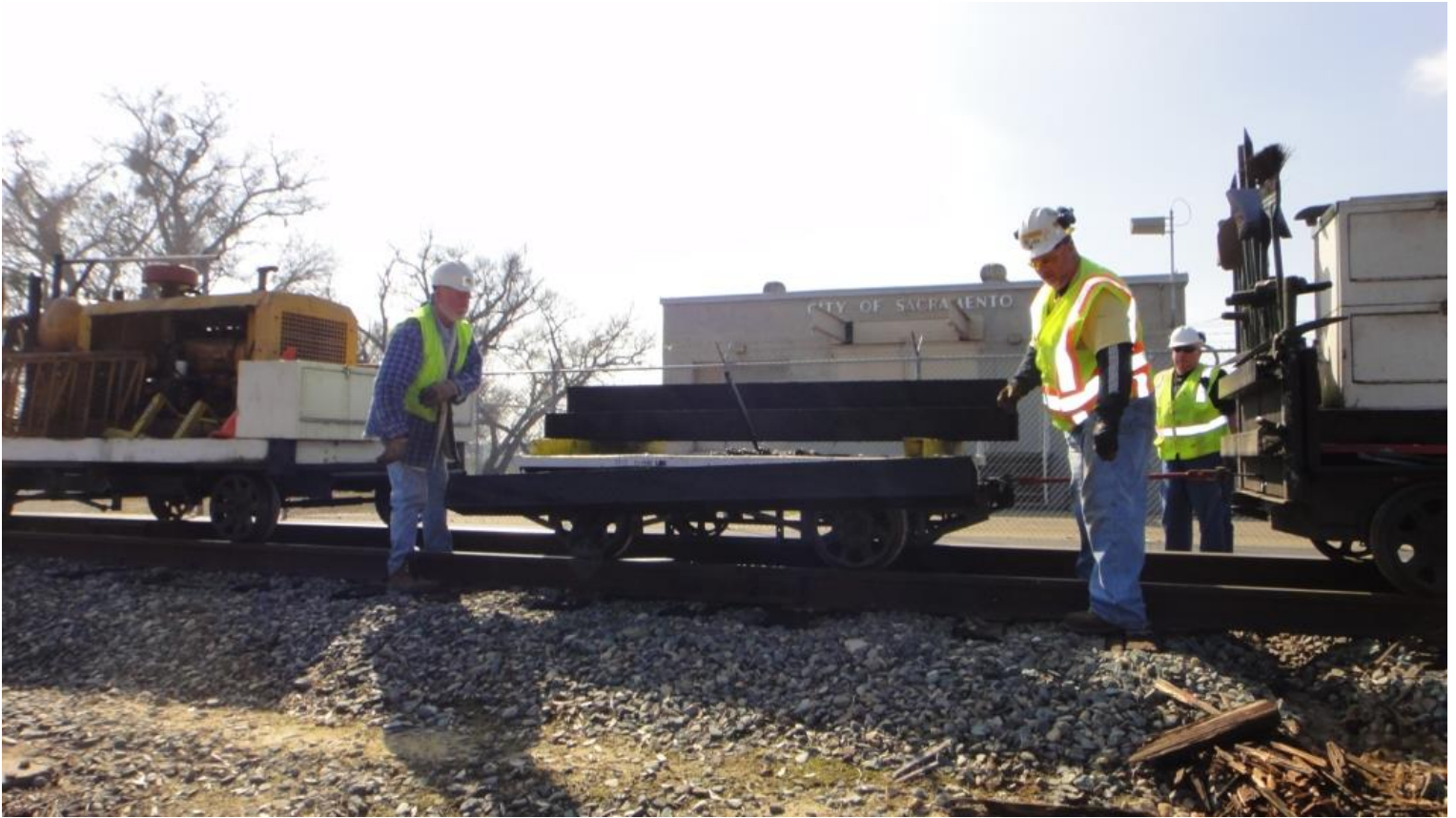
Mike M. and Mike F. toss new ties off the flatcar to replace those bad ties pulled by the 125
