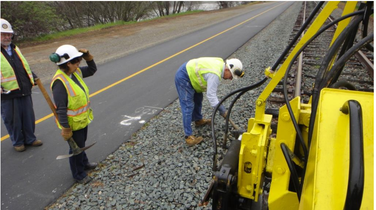
Pam takes a breather as Clem takes a turn at the mattocks digging out the end of a nasty tie
