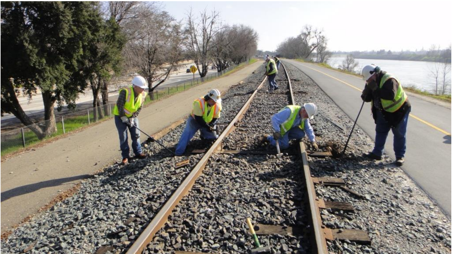
Three Mikes and a Frank: Mike W. nips-up the east end of the tie while Mike F. sets spikes. To the west, Mike M. sets spikes while Frank nips-up the tie.
